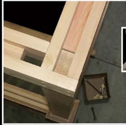
Top View of Beam / Post Connection
